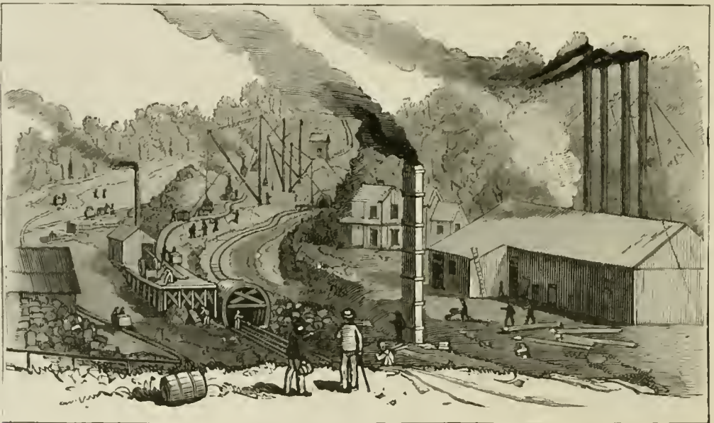
Fig. 12.—New Croton Aqueduct. Poantico Cut.
