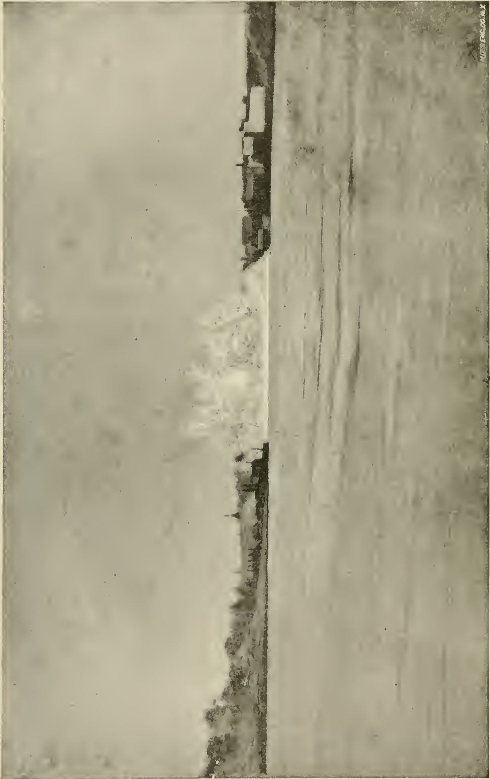
Fig. 1.—Explosion at Halletts Point, Sept. 24th, 1876. Area exploded, simultaneously, 2 \frac{3}{4} acres. Explosive used, 49,870 \frac{1}{2} lbs. Dynamite. Camera located 2,125 feet North-west of Explosion.
