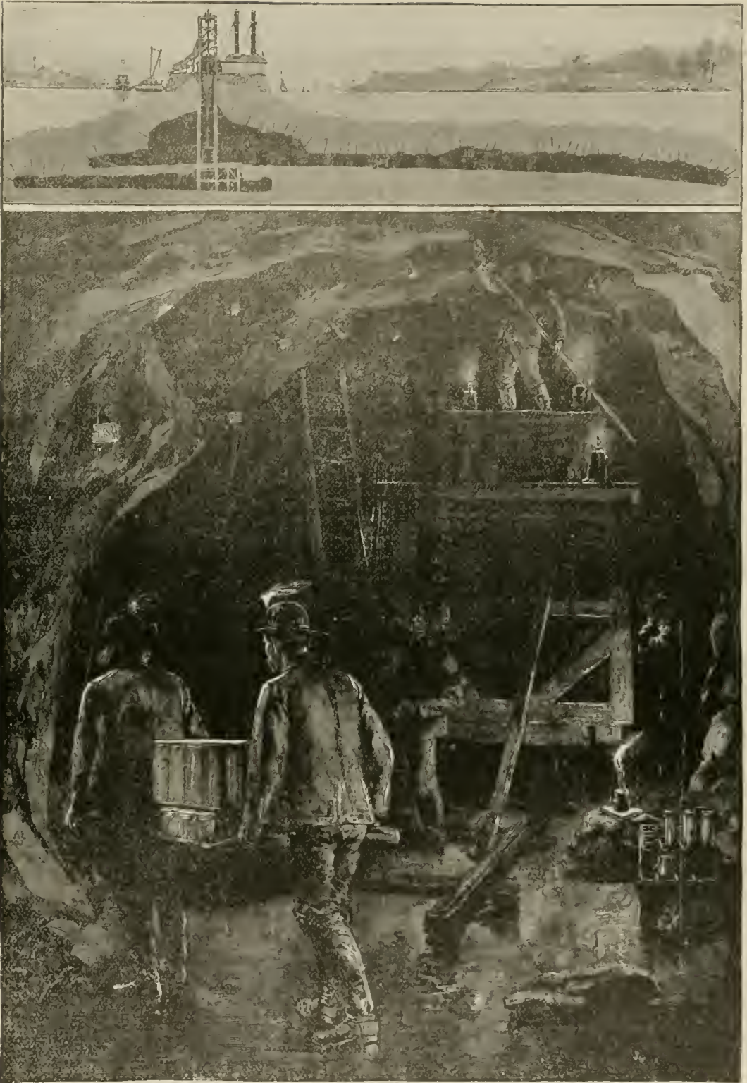
HIGH EXPLOSIVES. —Flood Rock. Interior view of Tunnel, showing the location of holes and method of loading them with the explosive contained in thin copper cases. After the holes are filled with Rackarock within a few inches of their mouths, a short case of Dynamite is inserted and left projecting to assist in producing explosion by "sympathy."
